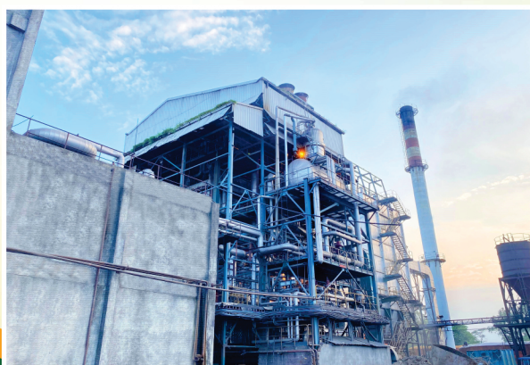
Works Location 4 : Village Lauhka, Teh. Patti, Distt. Tarn Taran, Punjab.
