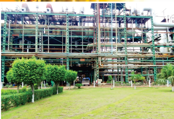
Works Location 3 : Village Karimganj, Teh. Shahabad, Distt. Rampur, Uttar Pardesh.
